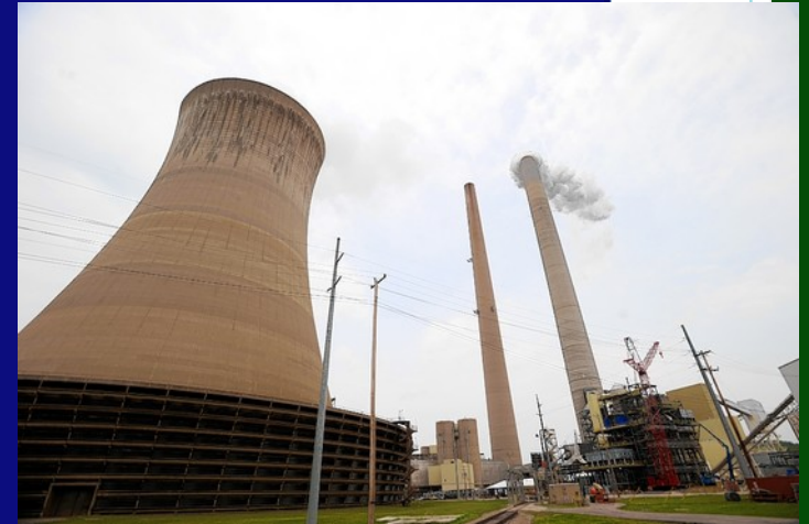
*Carbon Capture Component at Mountaineer Plant
